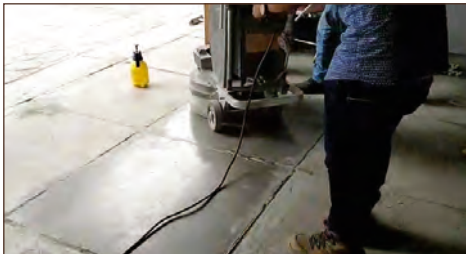
step 04 Polishing stage
