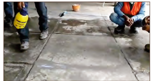
step 03 Liquid floor hardener
