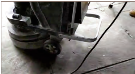
step 01 Grind existing concrete
