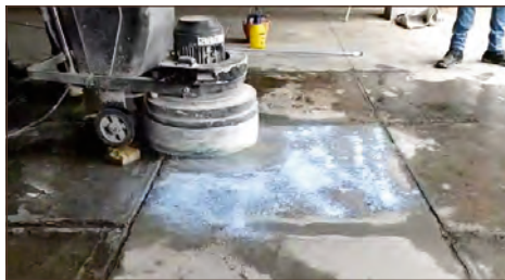
step 02 Crack reparations
